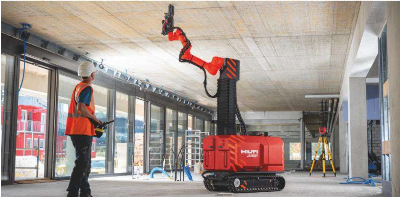
A BIM integrated robot scanning a building component
