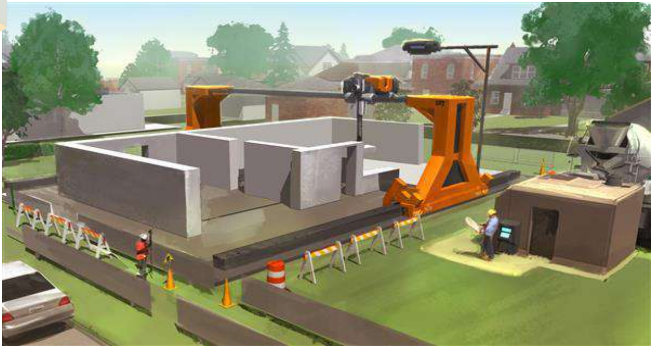
Render of a 3D printing construction process
