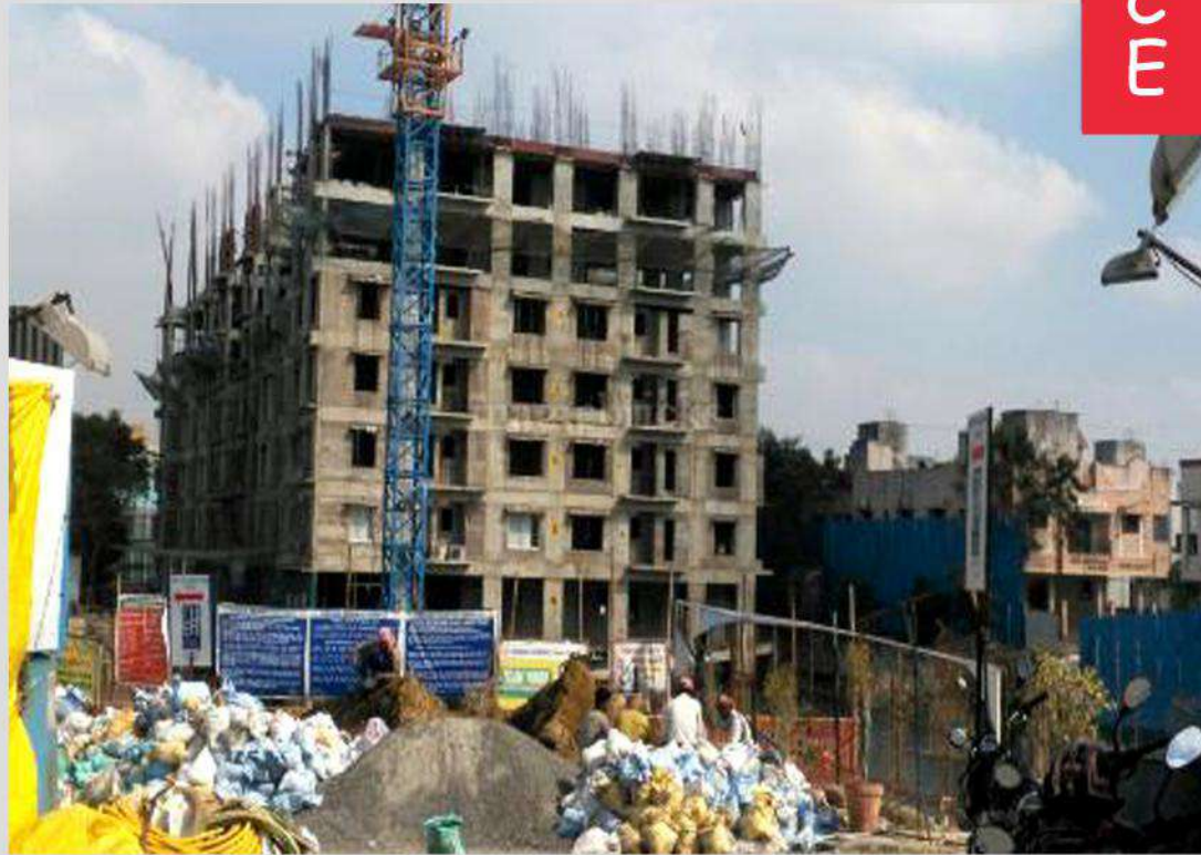
Esthell Golden Square Construction, Velachery
