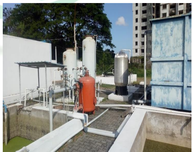
Figure 31: Sludge treatment plant (STP) in the campus
