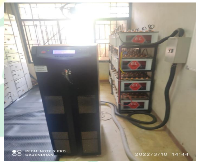
Figure 29: UPS's installed in the campus
