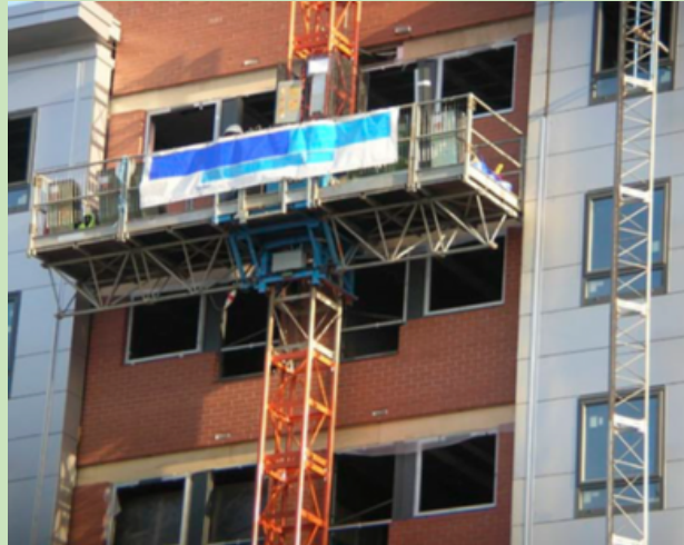
Figure 4 Mast climbing work platforms
