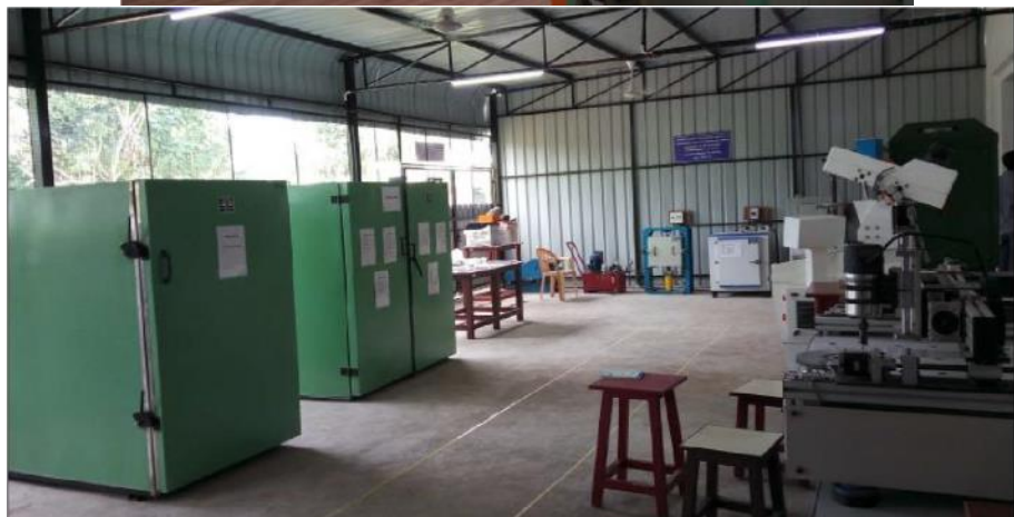
Figure 20: Coated Abrasive Disc Manufacturing Unit
