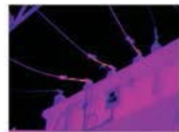
IR image of a high-voltage power line connected to a 115-23 kV substation Transformer.
