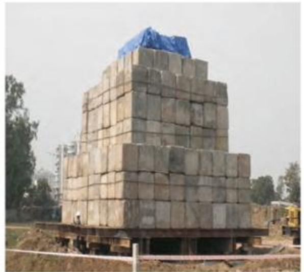
Static load test
