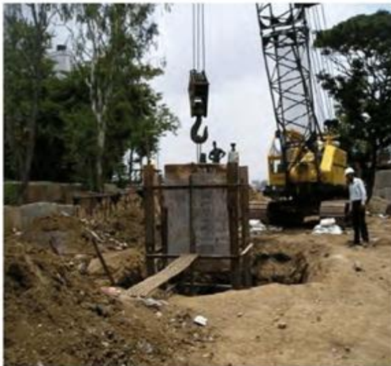
Dynamic load test
