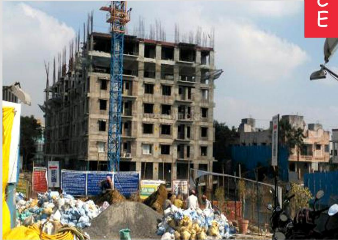
Esthell Golden Square Construction, Velachery
